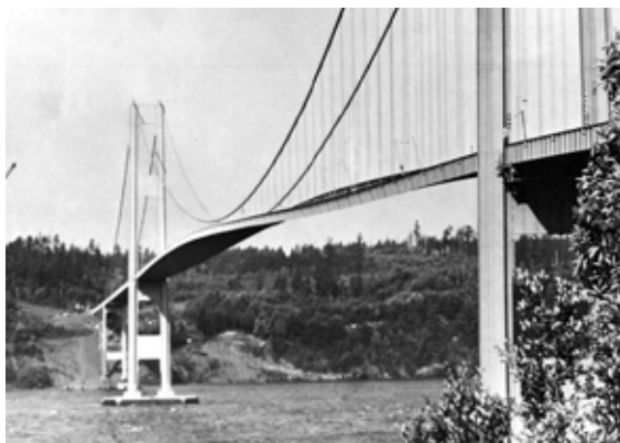
Tacoma Narrows Bridge
